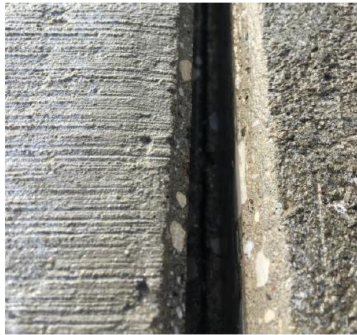
Figure 2 Photo of Wet Saw Joint Condition After Power Washing and Vacuuming
