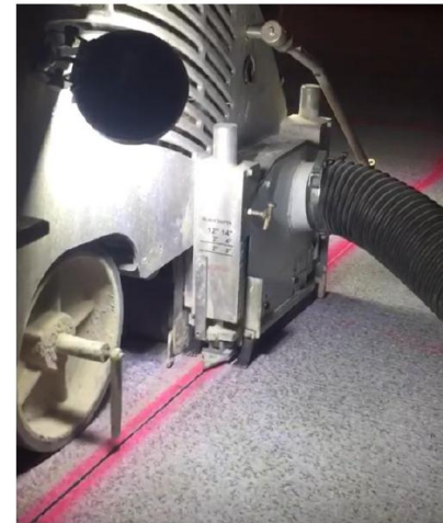
Figure 5 Photo of Early Entry Saw Joint With Vacuum Attachment
