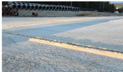
Figure 3 Photo of Concrete Remains from Early Entry Sawing without Vacuuming
