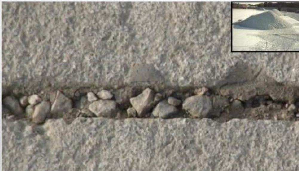
Figure 2 Incompressibles Accumulating in Joint During Construction
