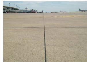
40-year-old Preformed Compression Seal at DFW Airport.
