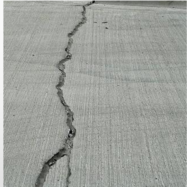
Uncontrolled Cracking
