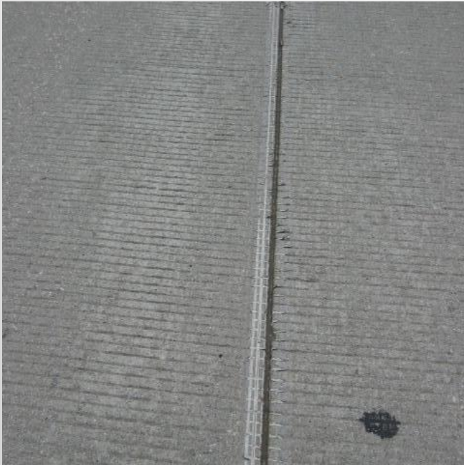
Controlled Cracking
