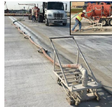
Figure 1 Photo of Wet Saw Vacuum Pickup Equipment
