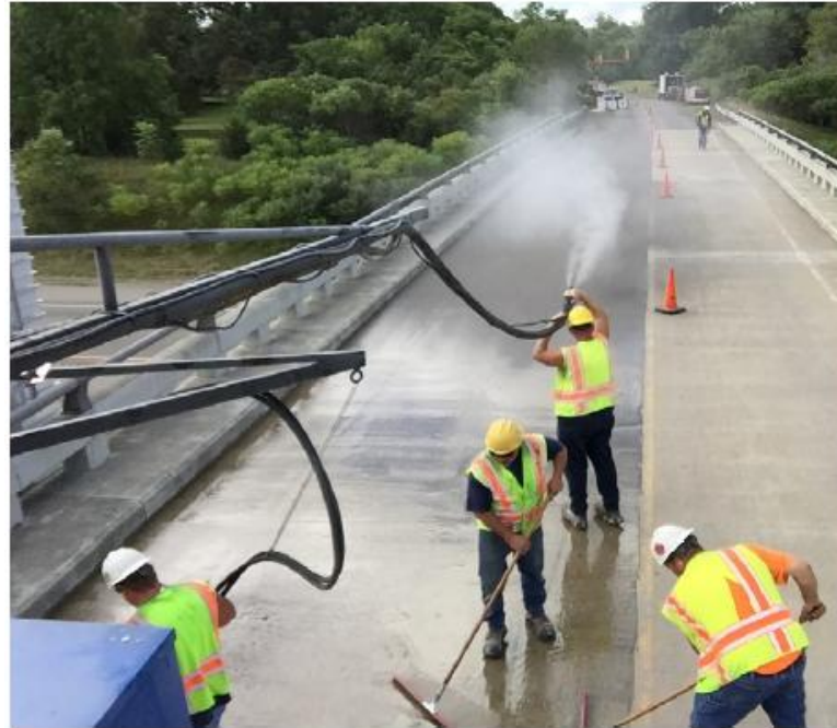
Figure 4. Broadcasting aggregate on sealer.
