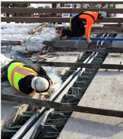
Figure 8. Joint replacement.
