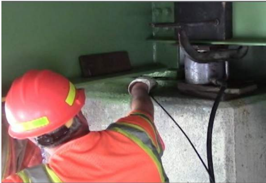
Figure 8 - Bearing Lubrication. Source GPI.
