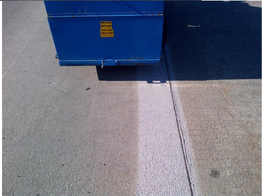
Surface Preparations: Shot blasting
