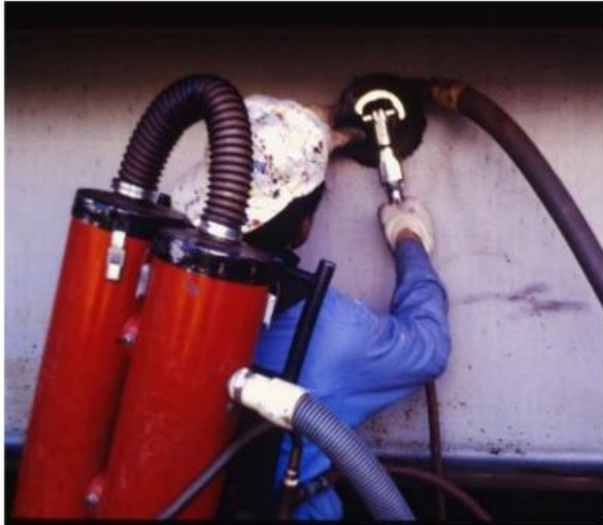
Figure 24. Shrouded grinder with back pack vacuum (pneumatic powered)
