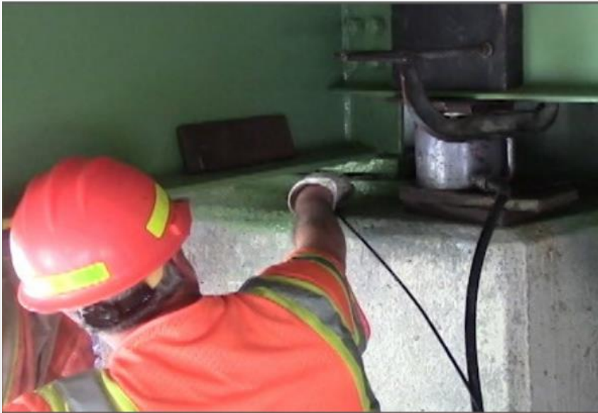
Figure 8 - Bearing Lubrication. Source GPI.
