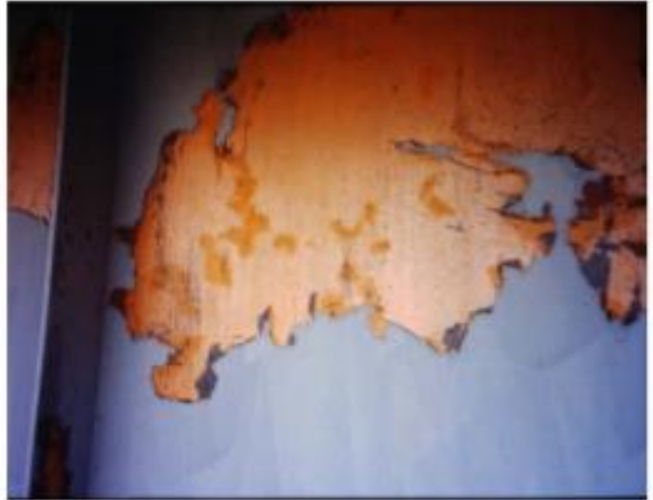
Inter-Coat Failure
