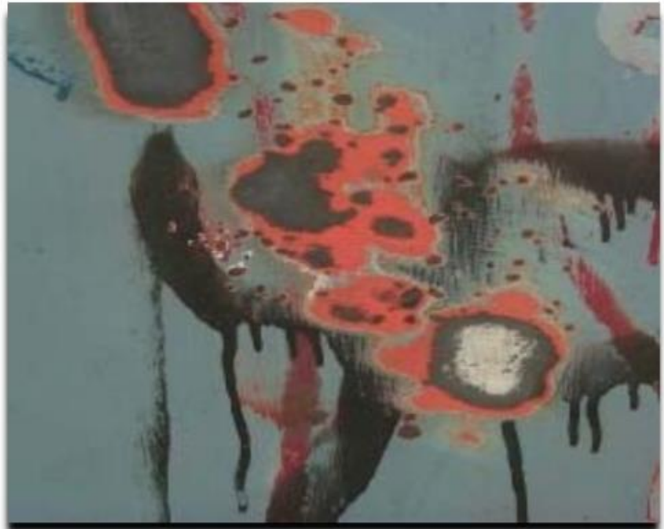
Figure 25. Feathering of existing coating
