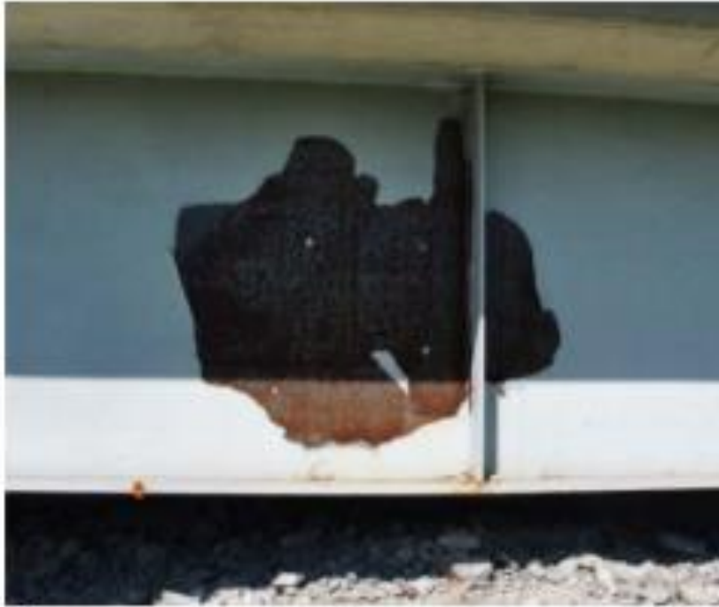
Coating Failure Exposing Rusted Mill Scale
