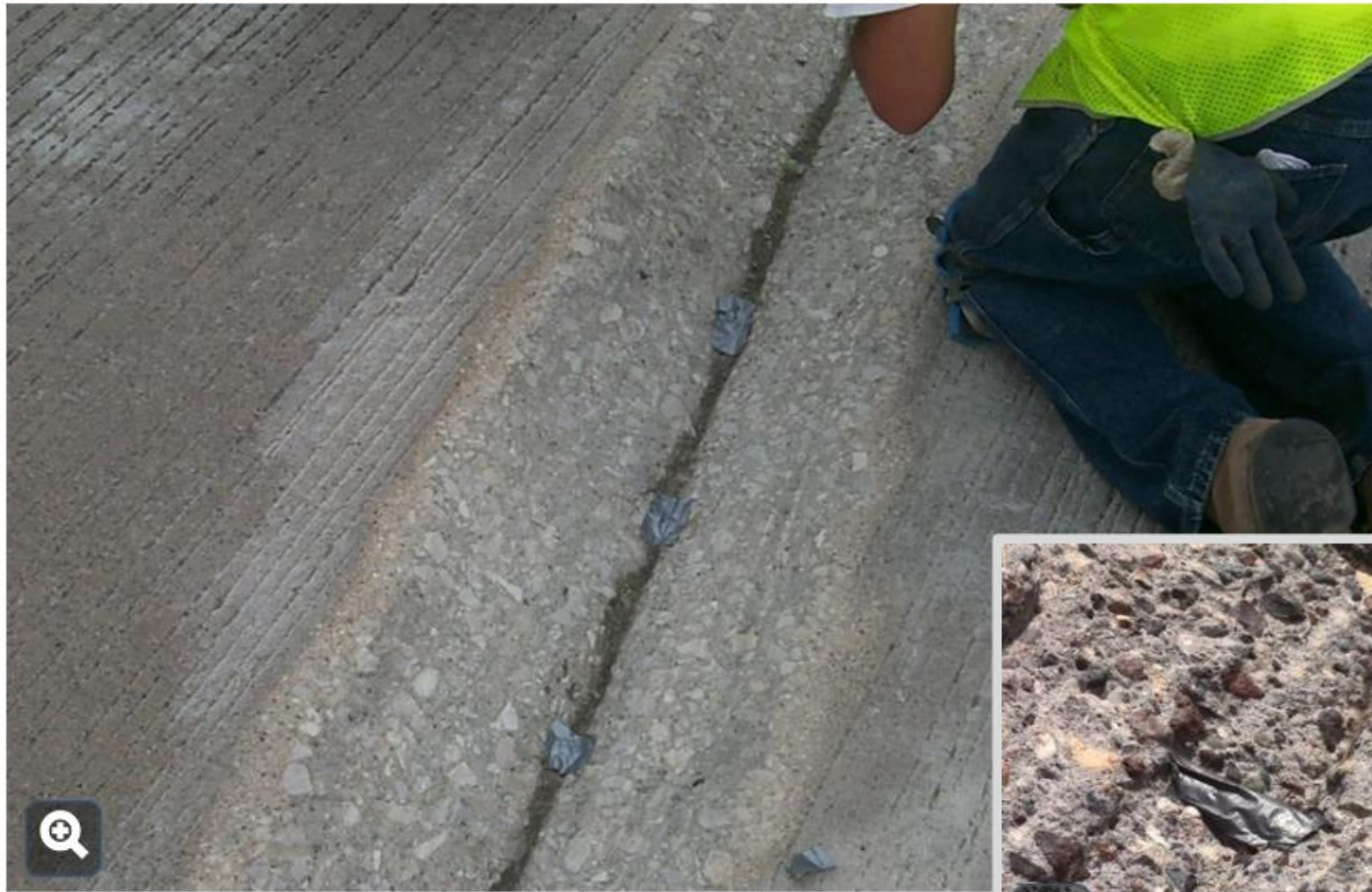
Applying duct tape to exposed dowel bars
