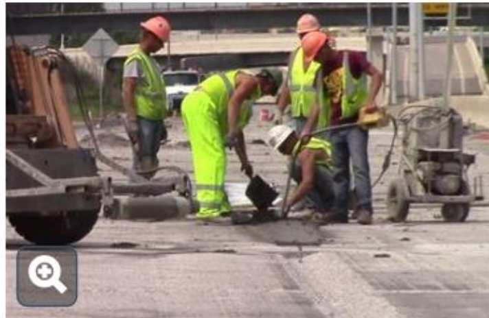
Placing, vibrating, and finishing 3U18 concrete patching mix
