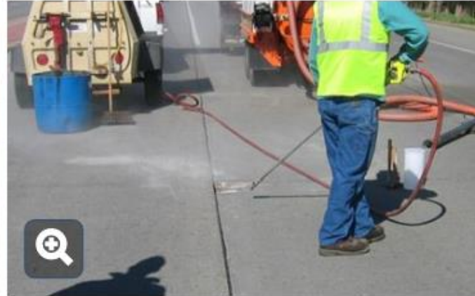
Maintenance crew using compressed air for final cleaning.
