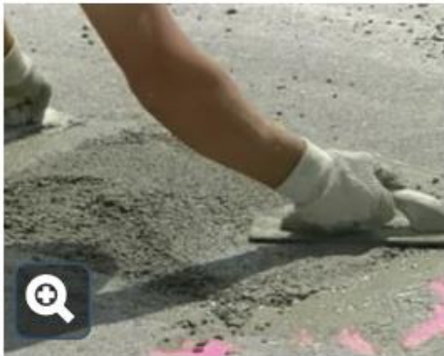
Close up of finishing partial depth repair
