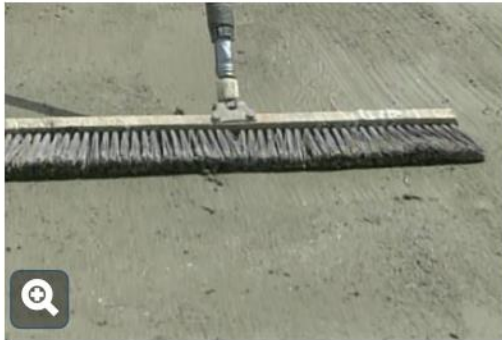
Broom texture for skid resistance
