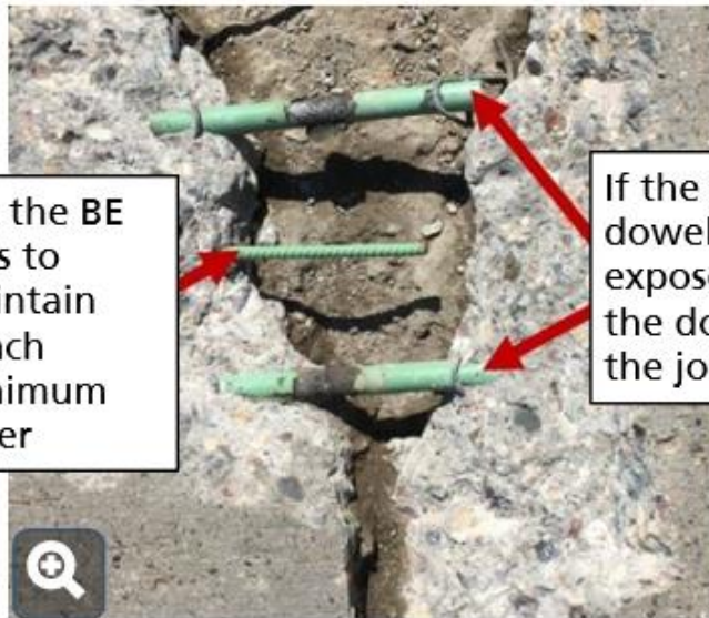
BE bars should not cross a transverse contraction joint
