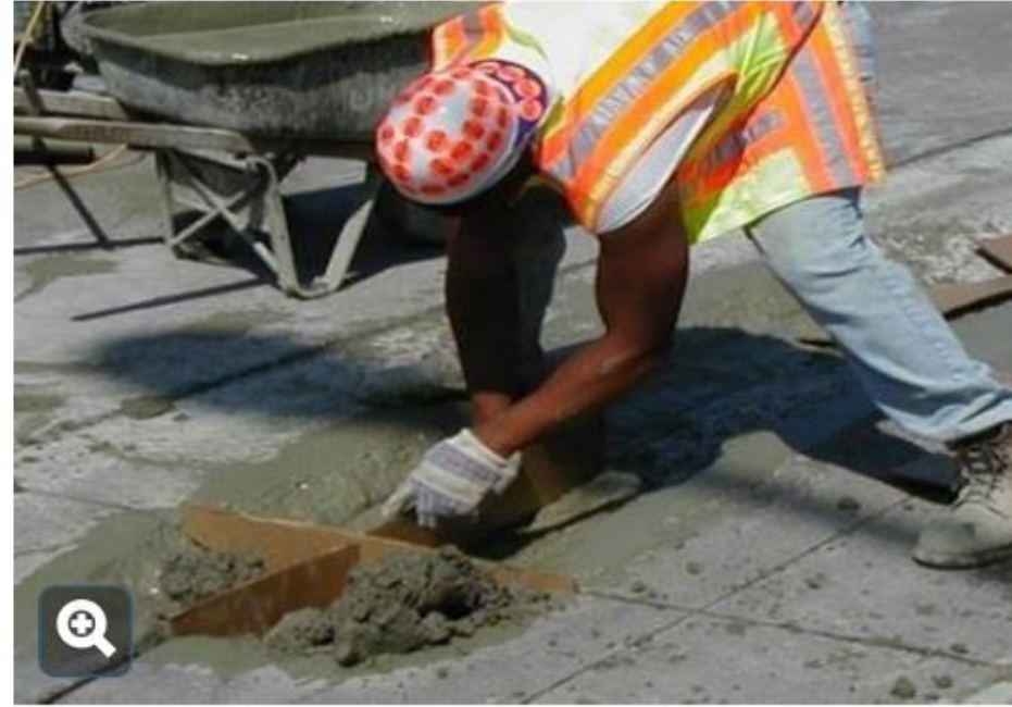
Re-establishing both transverse and longitudinal joints using wax coated cardboard
