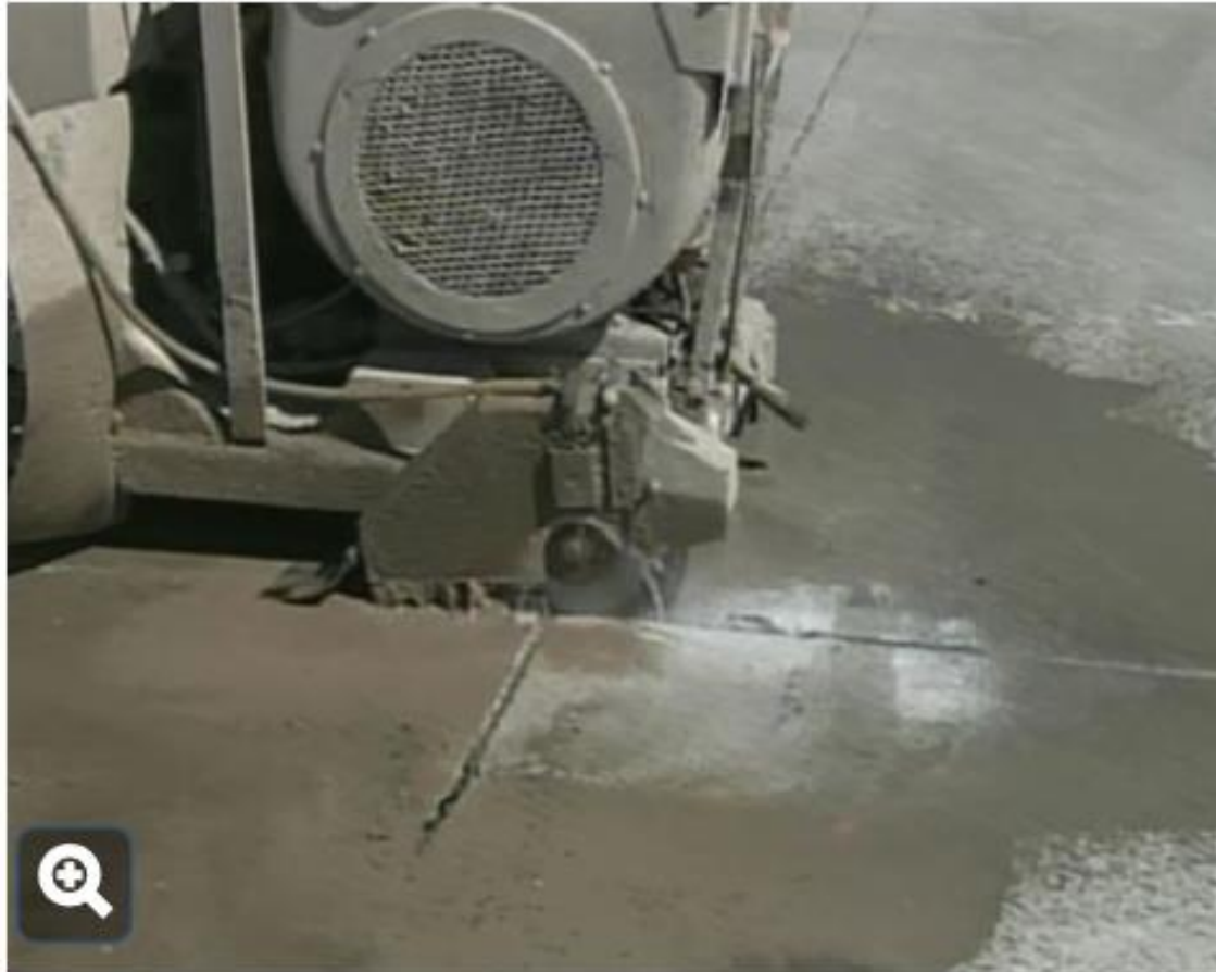
Sawing a Type B Repair
