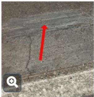
Sacrificial grout layer over taper edges one year later.
