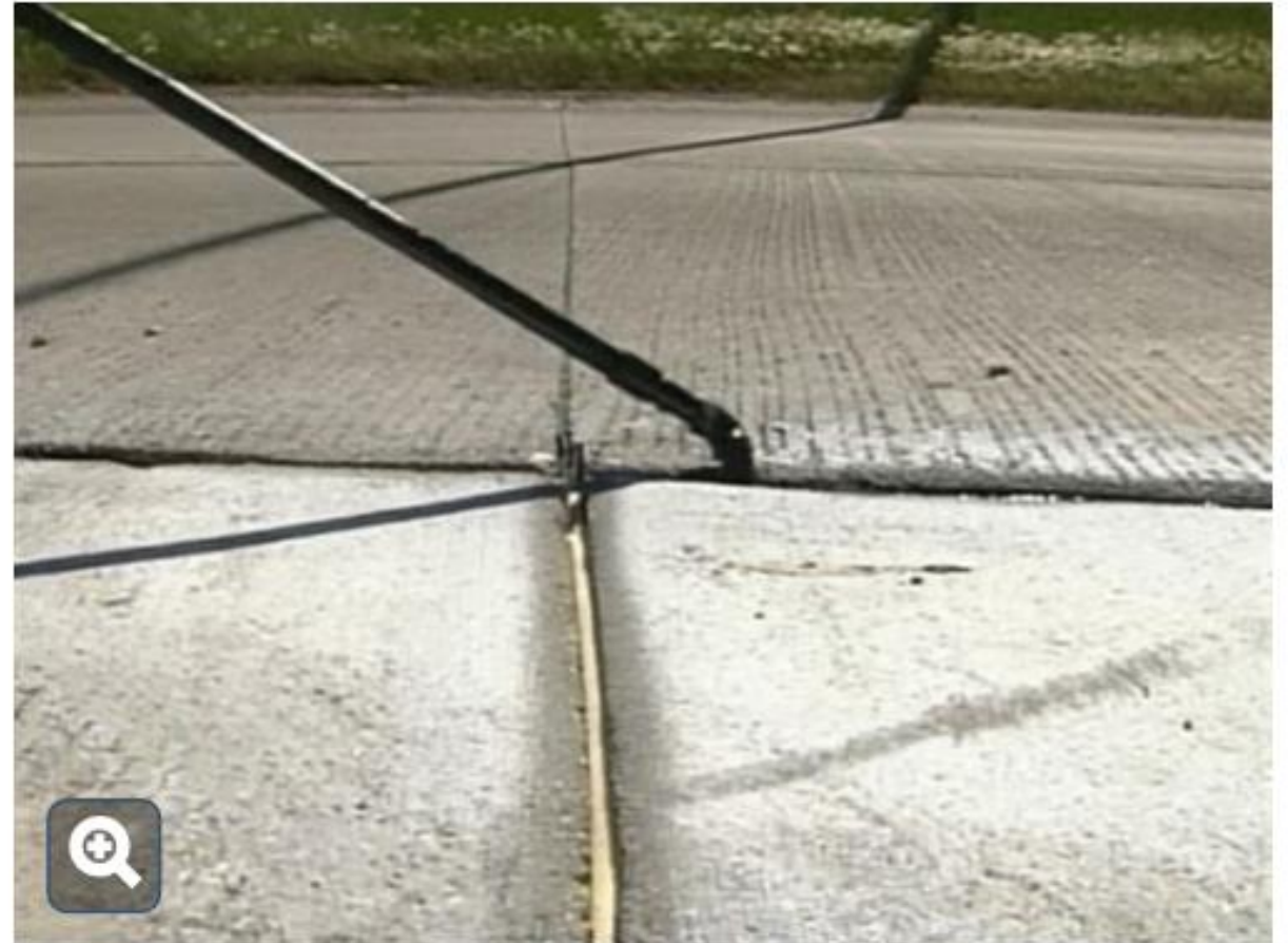
Sealing along a Type B repair
