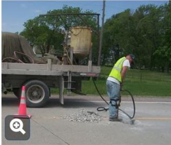
Chipping hammers are used for concrete removal below mid-depth of pavement ( t/2 )
