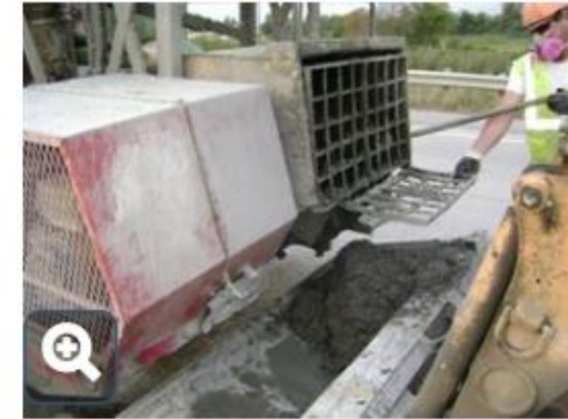
Back of truck concrete mixer for pre-bagged 3U18 mixes
