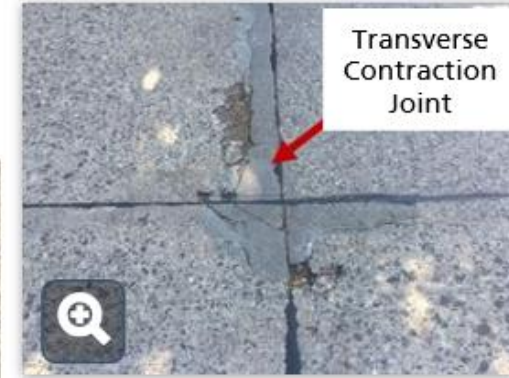
Transverse Contraction Joint
