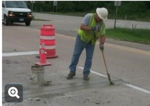
Applying sacrificial grout layer over tapered edges
