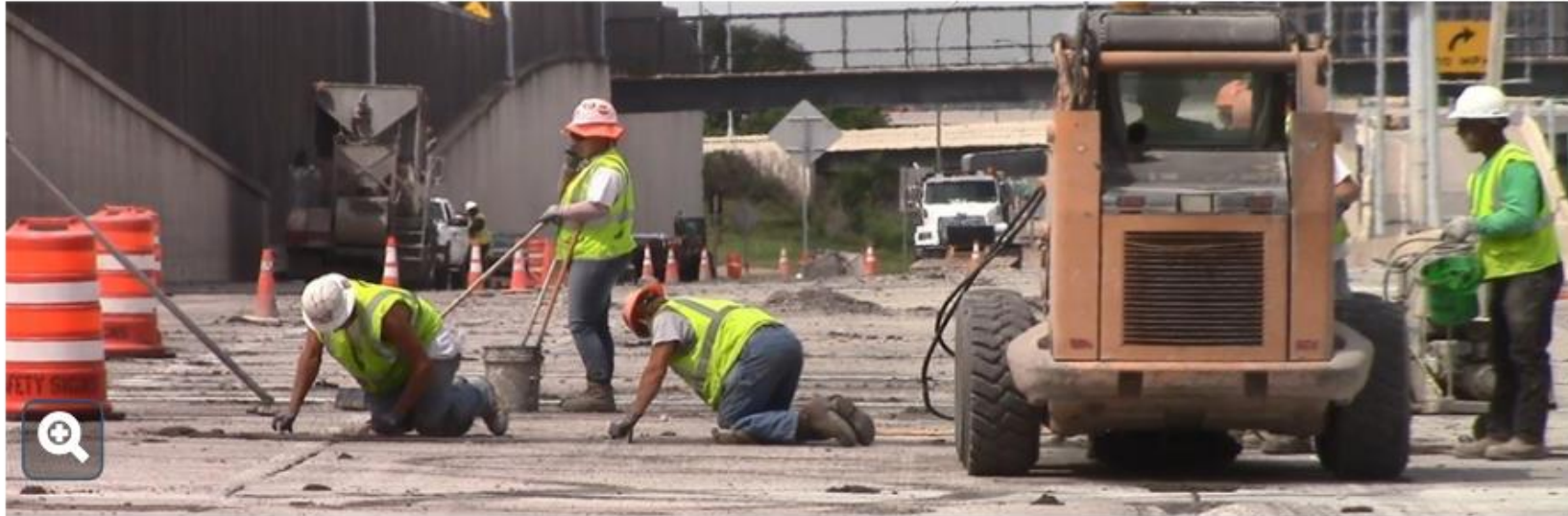
Finishing and edging partial depth repairs.
