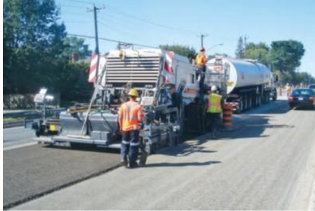
Single unit train with attached screed
