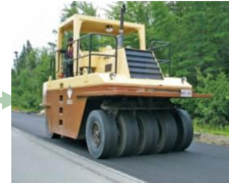
Compact to target density
