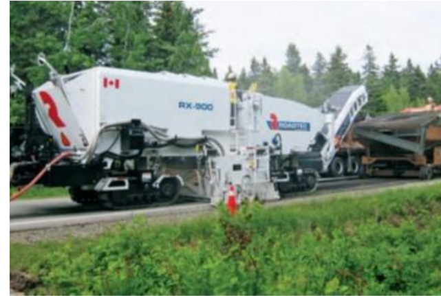
Feeding into scalping screen and hopper
