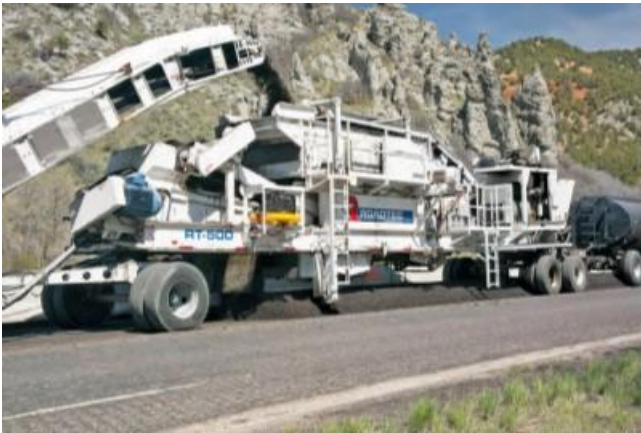
CIR crushing/screening unit and pugmill
