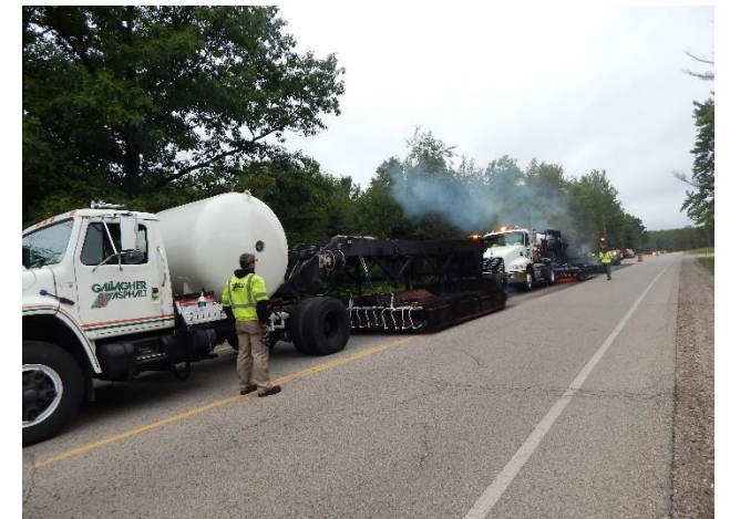
PHOTO: Dickinson County Road Commission
