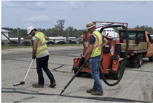
PHOTO: Dickinson County Road Commission
