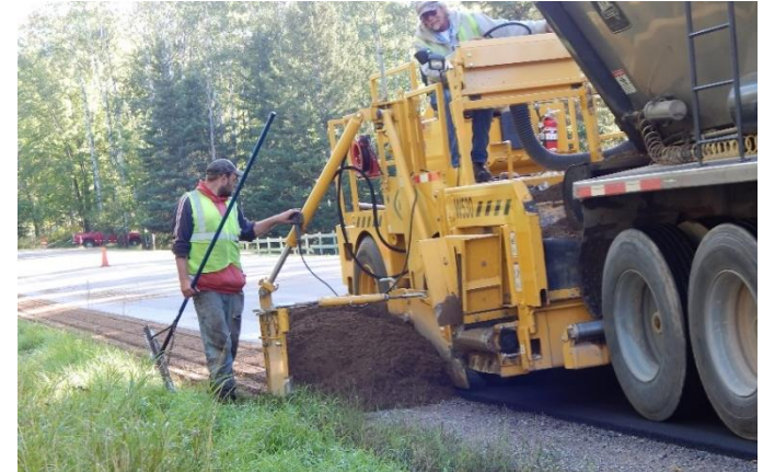
PHOTO: Dickinson County Road Commission
