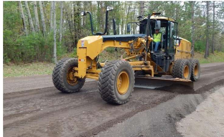
PHOTO: Dickinson County Road Commission
