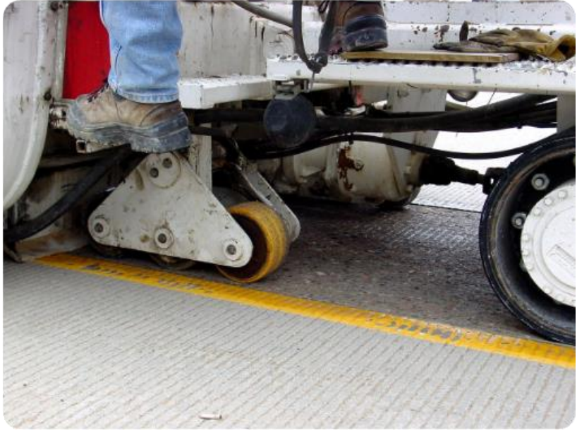
Proper Slurry Recovery System
