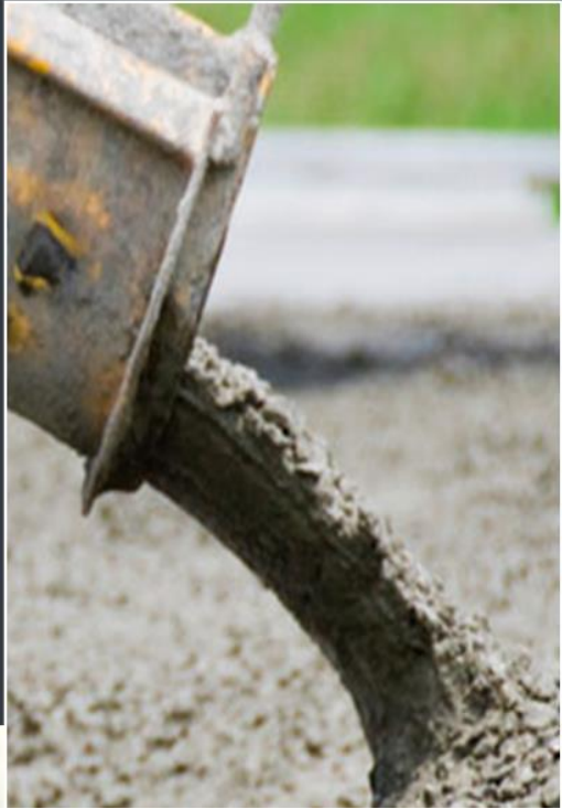
■ Step 1: Place Concrete
