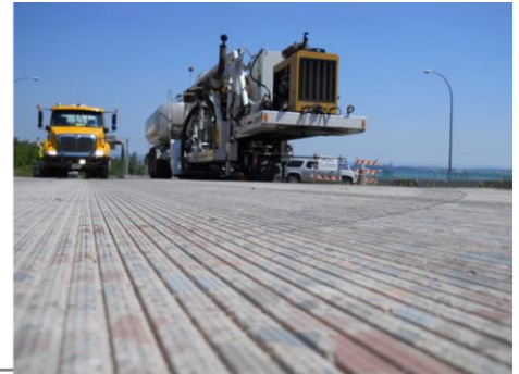
Next Generation Concrete Surface Or Grind and Groove
