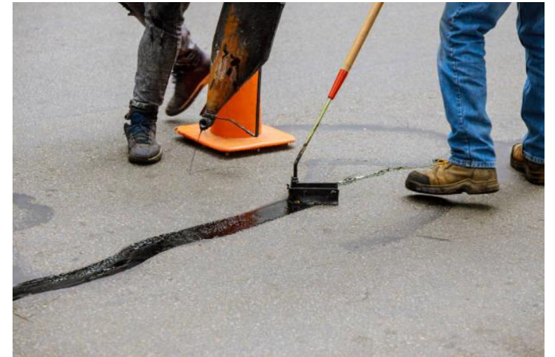
Typical Crack Sealing Operation
