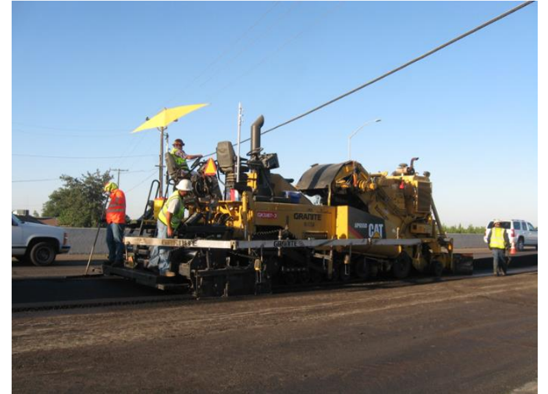
Thin Hot Mix Asphalt Overlay
