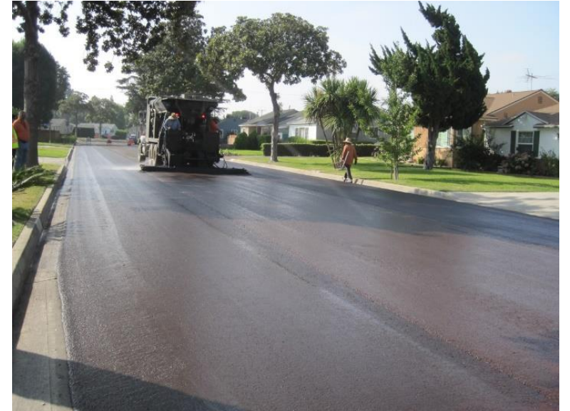
Typical Slurry Seal Construction
