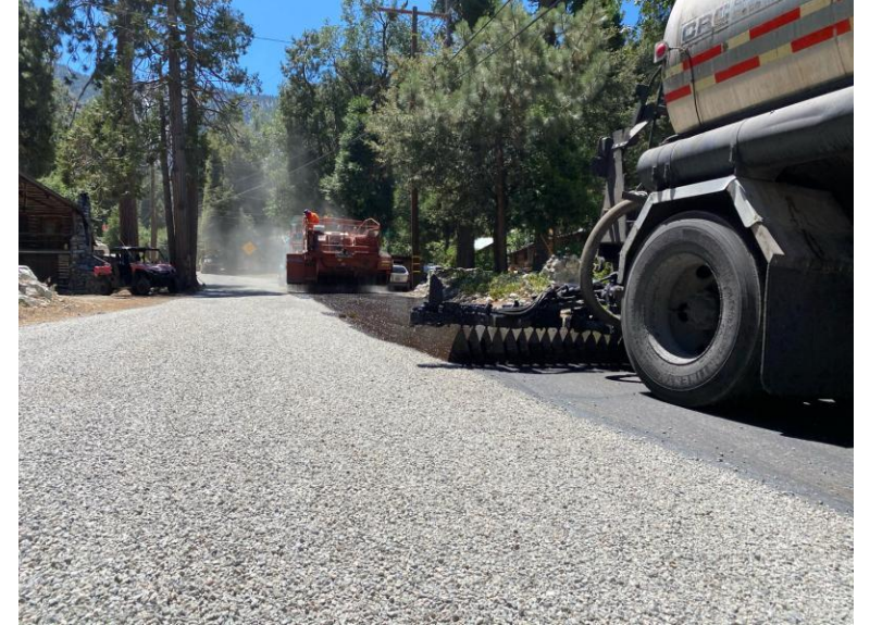
Typical Chip Seal Operation
