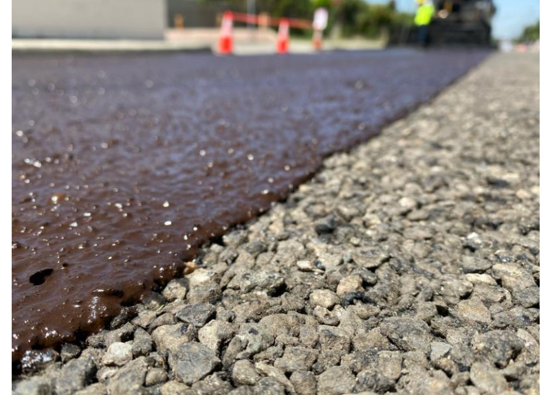
Completed Cape Seal - Slurry Seal over Chip Seal
