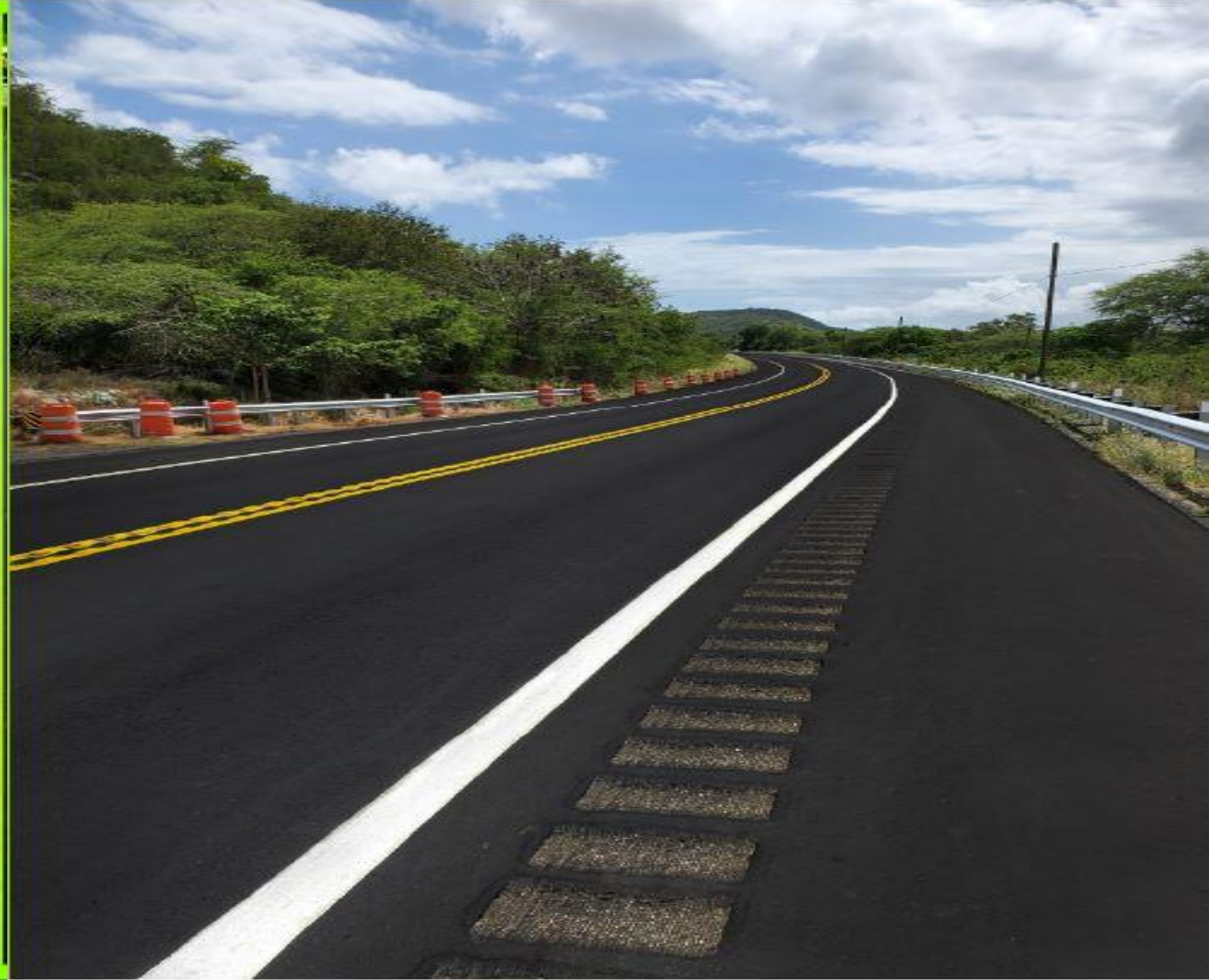
AFTER 2 LAYERS OF MICROSURFACING TYPE II
