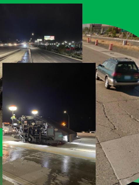
Thin Overlay on Concrete (Ultra-Thin **Bonded Wearing Course)** Done many UTBWC projects in Las Vegas with spray paver and modified emulsion tack coat Highly Modified Asphalt (PG70-34NV) Application on PCCP subjected to freezethaw First project on I-80 has been awarded Second project on I-580 in Reno has been placed!!
