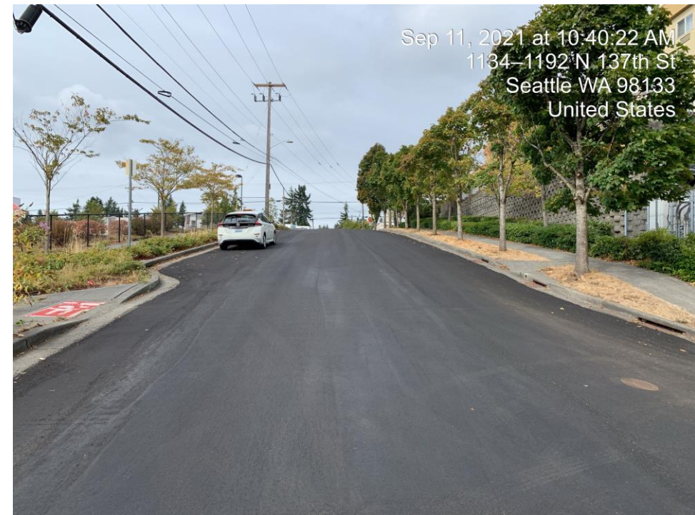
1100blk of N 137 th St - After Slurry Seal
