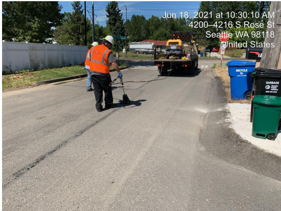
Preparing Cracks for sealing
