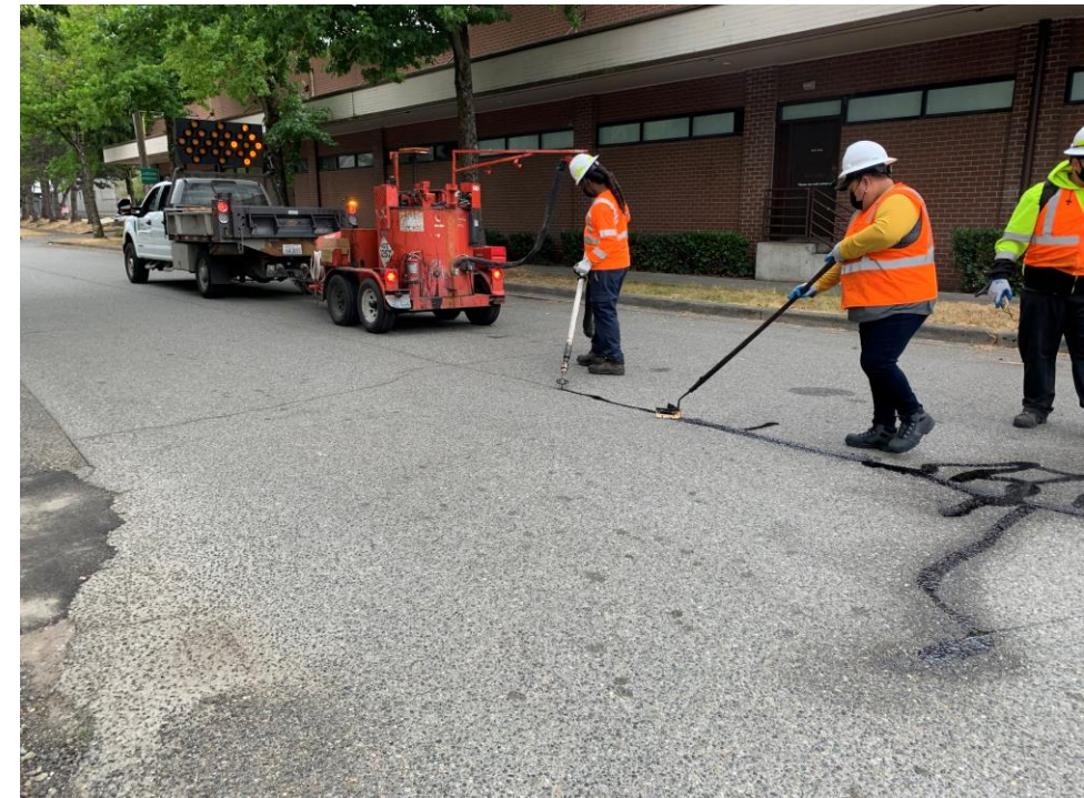
Sealing Cracks
