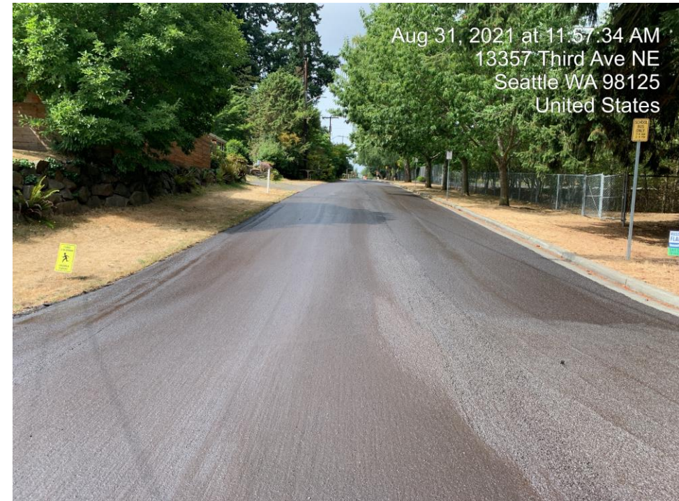
200blk of NE 135 th St - After Slurry Seal
