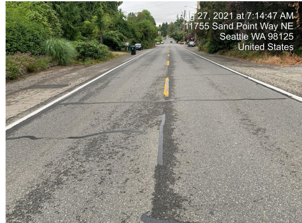
11700blk of Sand Point Way NE - After crack sealing
