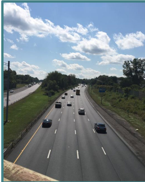
Mill and Overlay
