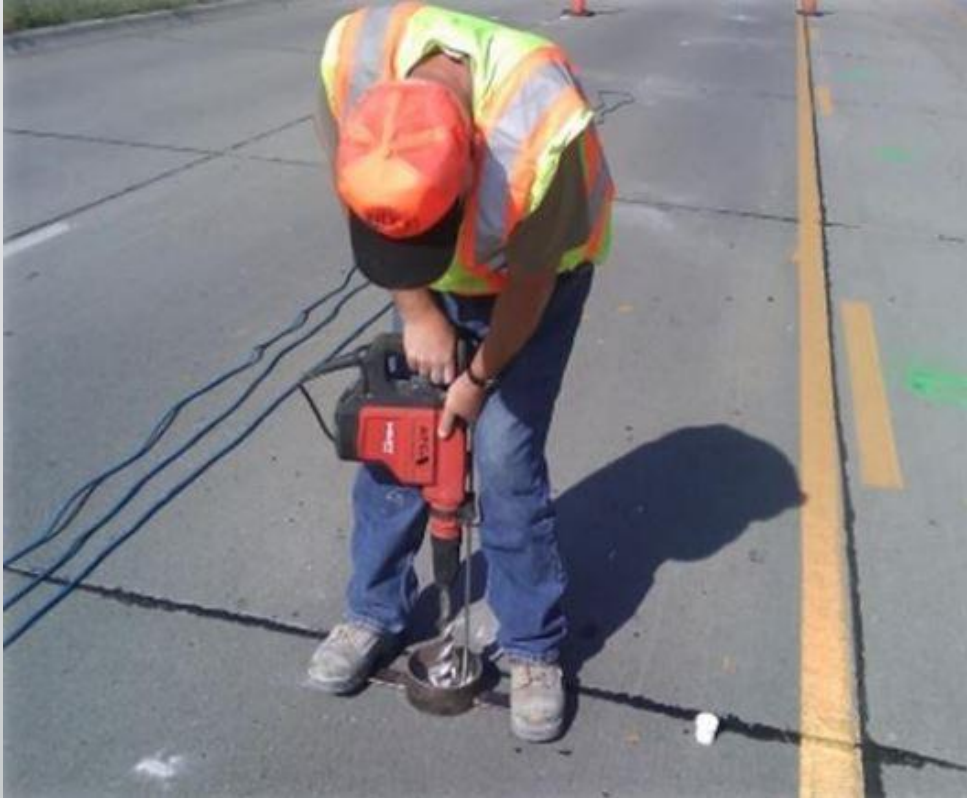
Drilling for Chloride Ion Sample
